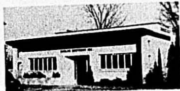
New Quarters for Buhler Brothers milling machinery division at 4207 Nicollet Avenue, Minneapolis, Minnesota.
